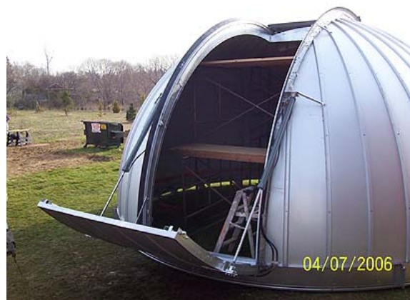
The completed dome awaits the crane
