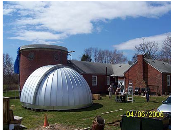
View looking southwest with completed dome in the foreground
