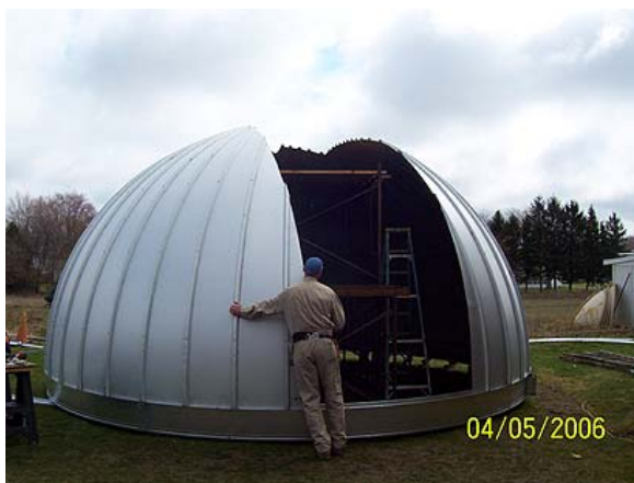
Jim inspects the partially completed dome.
