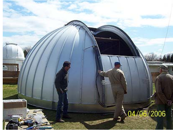
Lower section closed with the top section open and fully retracted at the crown
