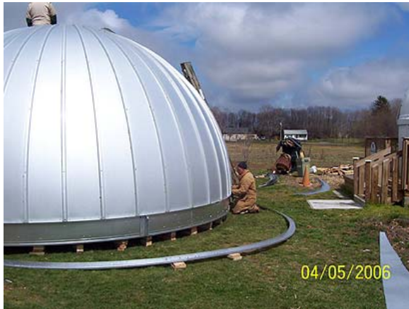
Larry works on securing the rim and base of the dome.
