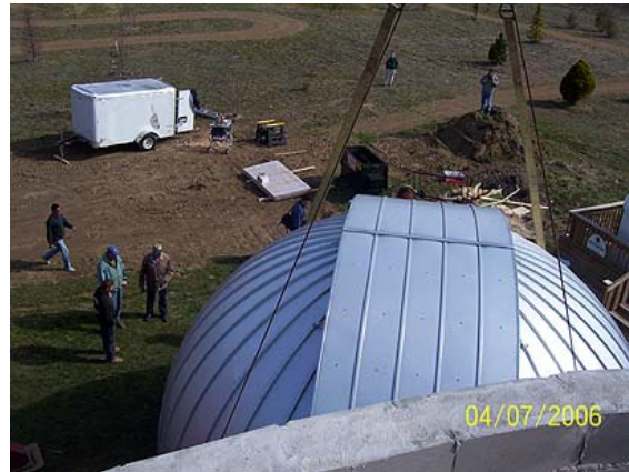
The completed dome being hoisted up and out of the gravity well, on a one-way trip to a refurbished base rim
