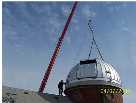
In a view looking northeast, we see David as he removes the sling bolts from their respective mounting points
