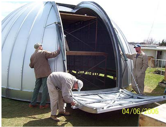
Shutter fully open, showing the lower, hinged section opened out with the top section fully retracted at the crown
